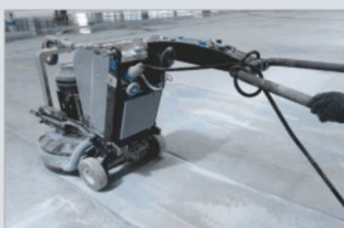
Floor grinding equipment
