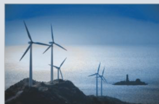
Wind power generation
